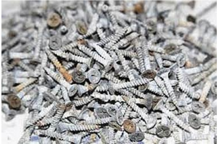
The beginning stages of rust formation on these zinc phosphate-coated metal screws demonstrate the limitations of using phosphate coatings alone in the prevention of corrosion.
